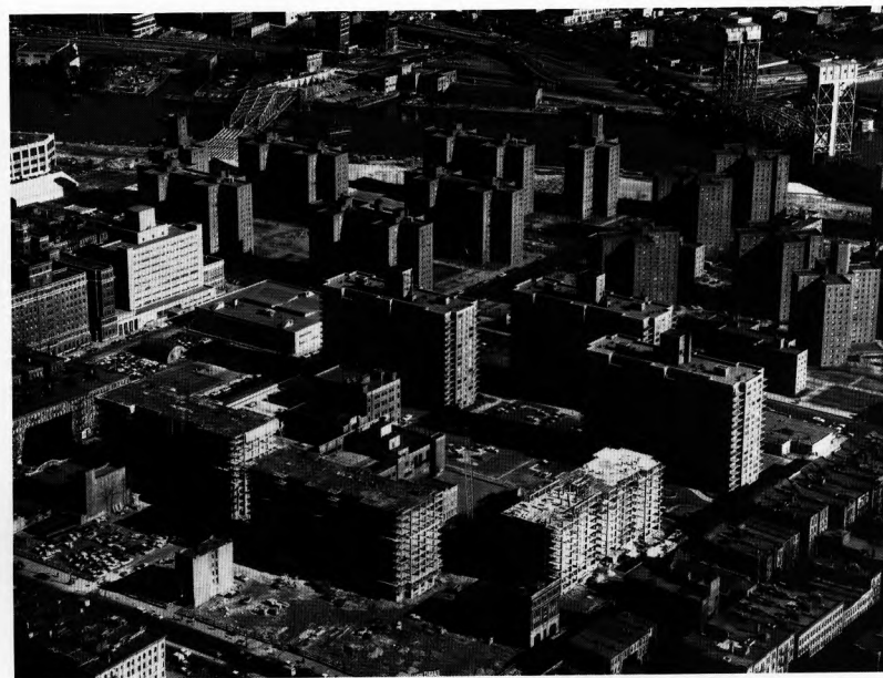
E-37. Lenox Terrace under construction (center), Abraham Lincoln Houses (cross-shaped towers at right), and Riverton Houses (double-cross slabs), early 1958. Fairchild Aerial Surveys, Inc.
