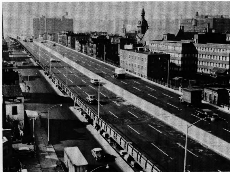
E-22. Brooklyn-Queens Expressway, ca. 1960
