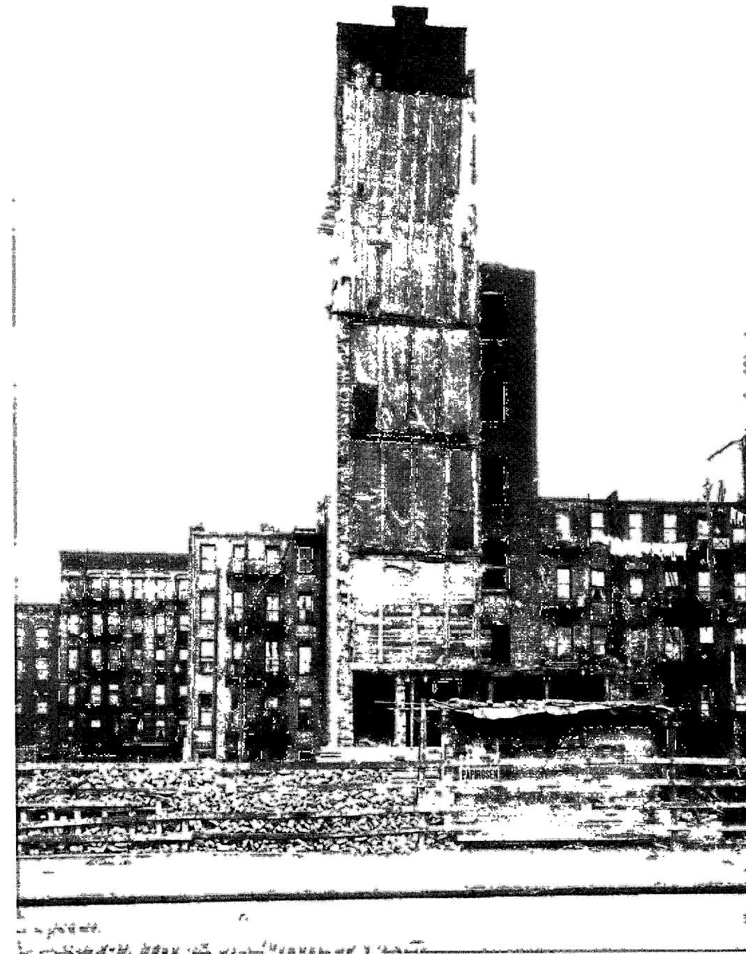
Fig. 3.14. A lone tenement on Essex Street between Stanton and East Houston awaits demolition to make way for the Essex Street Market, 1935. A quarter century later, similar images would be found throughout the Lower East Side, as public housing and slum clearance were embraced by city planners. Collections of the Municipal Archives of the City of New York.
