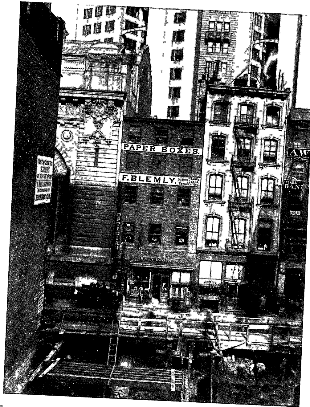
Fig. 1.4. George P. Hall, Construction of a Building . George P. Hall collection, 1902-1906. Museum of the City of New York.
